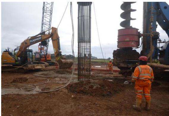
23-Feb-22: Pile cage being vibrated to position
