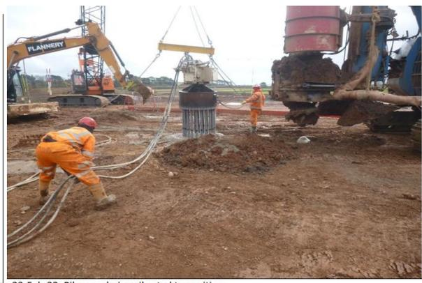
23-Feb-22: Pile cage being vibrated to position
